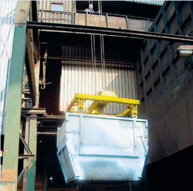
Bi-modular skips supplying the blast furnace
